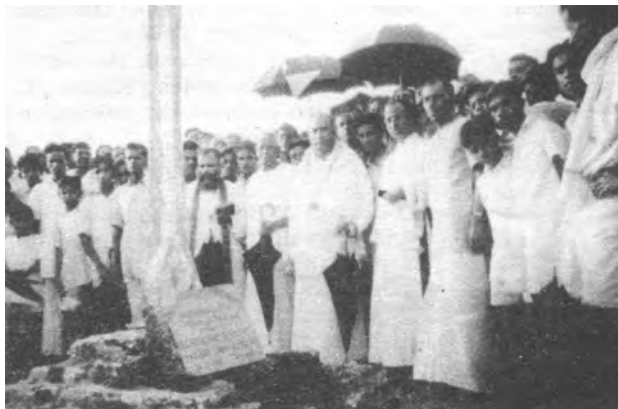
Laying foundation stone by M. O. Thomakutty trustee Rev. P. T. John Deacon M.O. Vargheese, stand- ing beside it.
